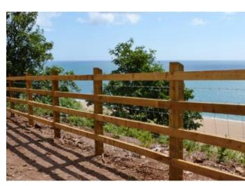
1.2m high timber post and rail fence to swales and drainage pond
