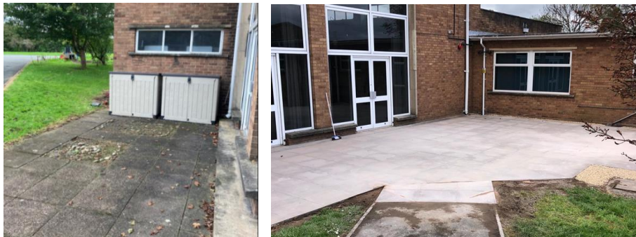
Before & After Photos of paving improvements at Donnington Wood Infant School
