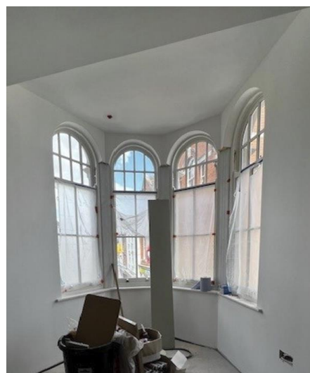
Interior restoration to Nuplace apartments
