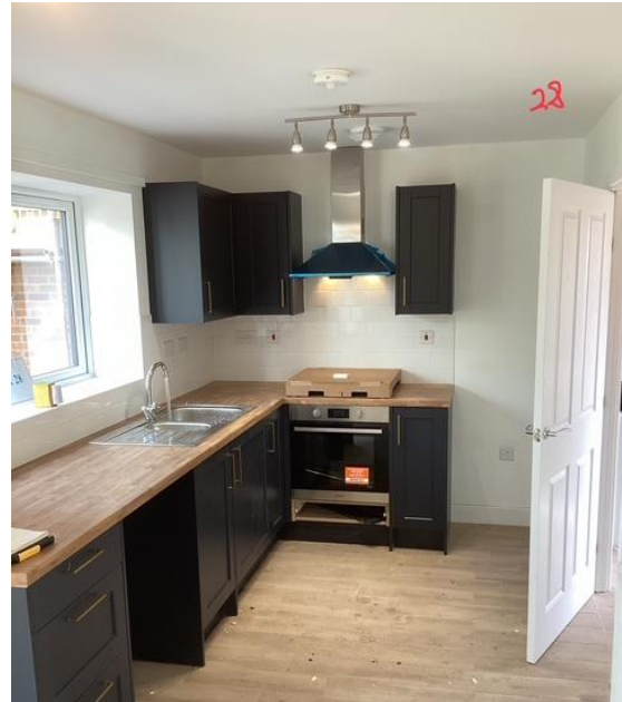
Internal kitchen fit out
