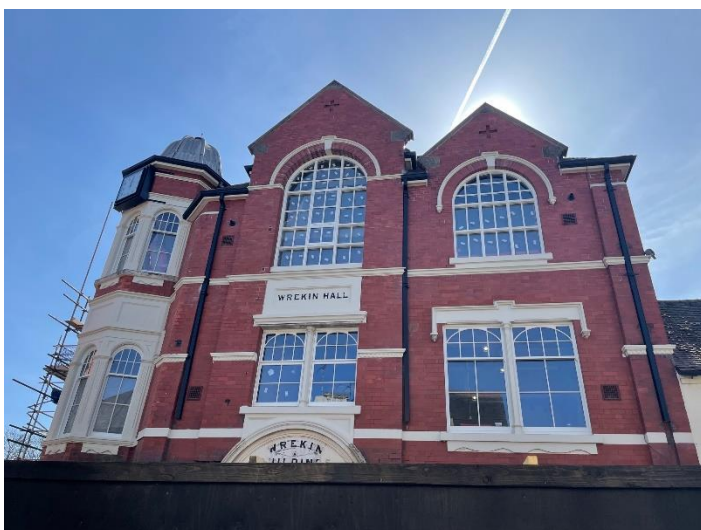
Exterior of the building post refurbishment
