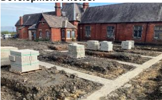
View: Rear of the building showing foundations to new build dwellings
