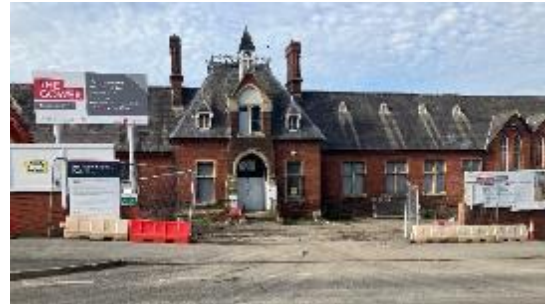
View: Front of building showing entrance widening
