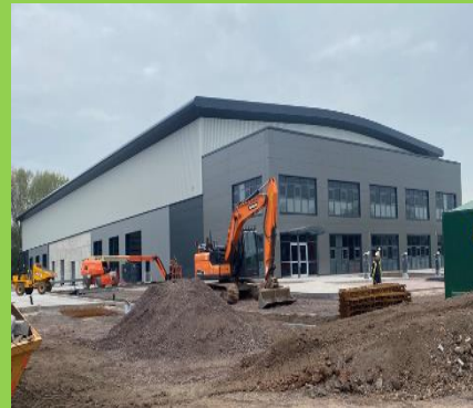
Hortonwood Plot 11e – Trebor – In progress
