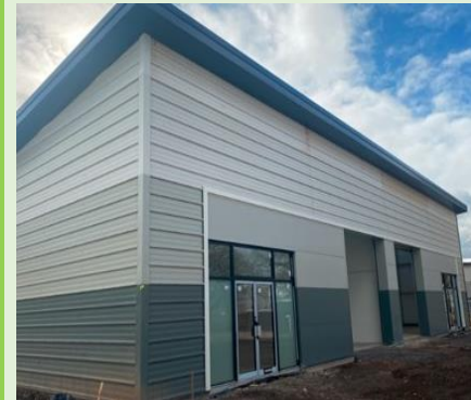
Hortonwood Plot 12 – TWC – In progress
