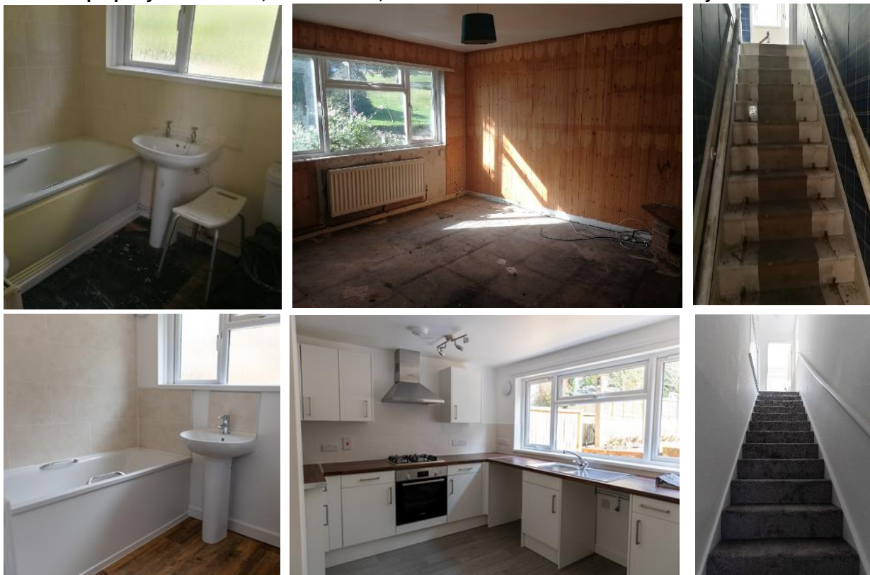
Photos of property in Sunnyside, Coalbrookdale, before and after refurbishment works by TWH
