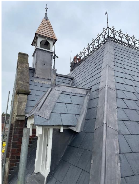
Intricate restoration of roof detailing.
