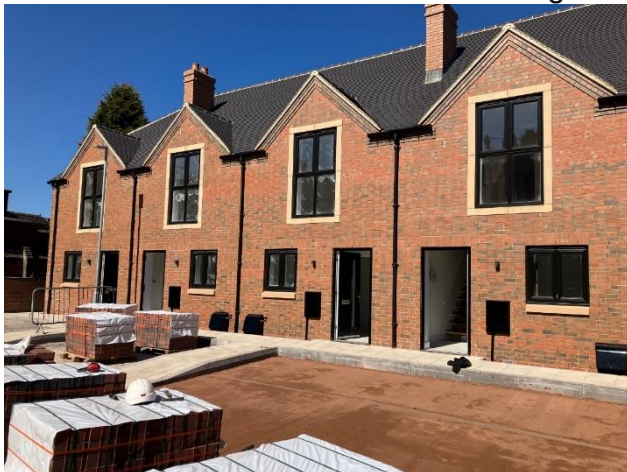
New build homes to rear of site
