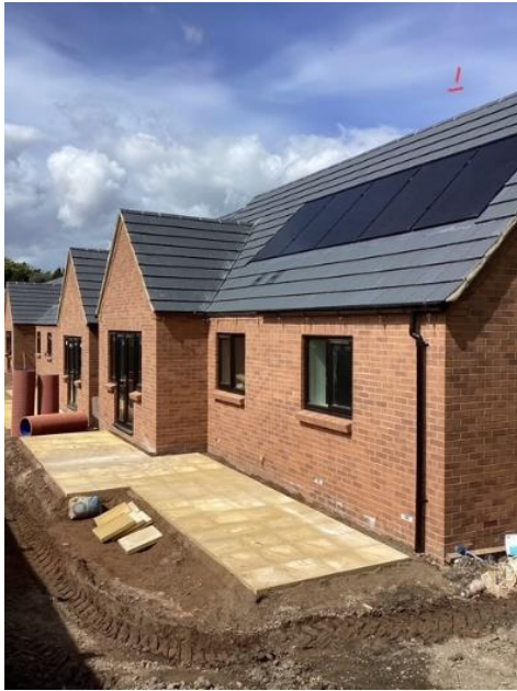
New build bungalows
