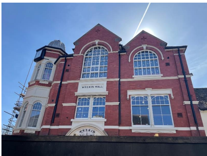
Exterior of the building post refurbishment
